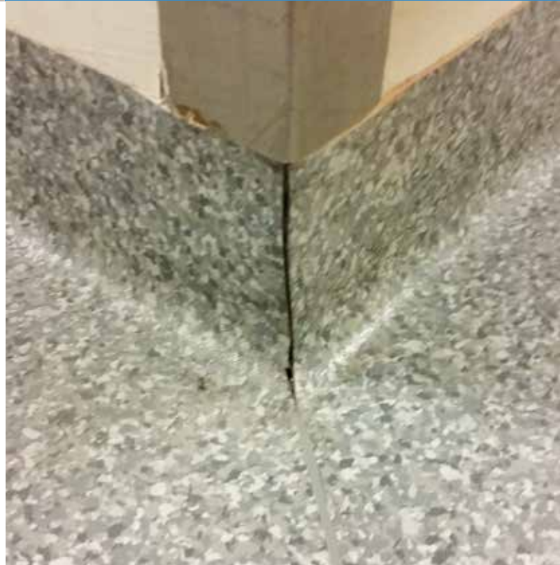
Outer corner fabricated by hand on site
